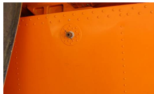
Level indicator Tank No. 3.
